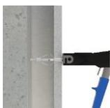
Place the bolt into the installation gun. Push the trigger until the anchor is fully expanded.
