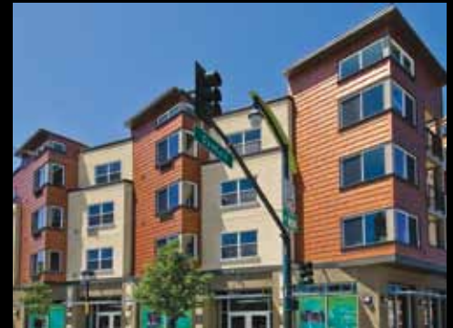
SAN FRANCISCO, CA Below Market Rate Development for first time home buyers. Located in the City's Bayview District, a community for those looking for the newest urban haunt. 4800ThirdStreet.com WEB: 0084837 $155,864-$272,934 Linda Harrison, 415.772.8452 San Francisco Brokerage
