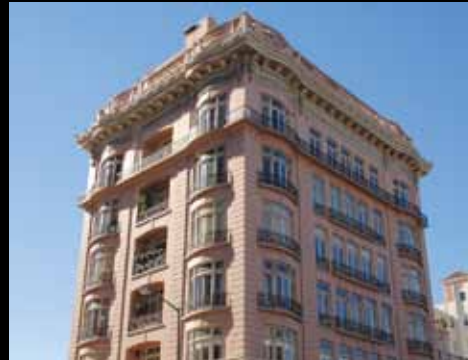
SAN FRANCISCO, CA Nob Hill: Extraordinary full floor atop SF's most beautiful Beaux Arts building. Living Room with stained glass skylight; Library & Den; Terraces with dramatic views; Air-conditioned; Doorman. PenthouseOnNobHill.com $3,500,000 WEB: 0084977 Gregg Lynn, 415.901.1780 San Francisco Brokerage
