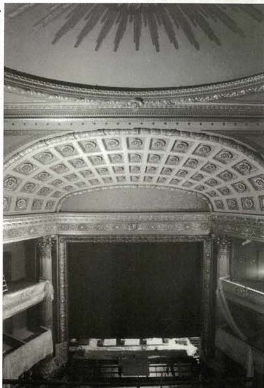
The 85-year-old Geary Theater, damaged in the 1989 Loma Prieta earthquake, reopens this month.
