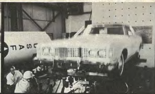
THEN: A million brutal shakes on Thiokol Laboratory's missile vibrator in Utah.
