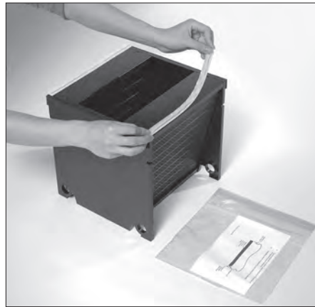
Step 3: Repeat to install the second butterfly gasket on the other side of the leaving air side face of the half-cassette.
