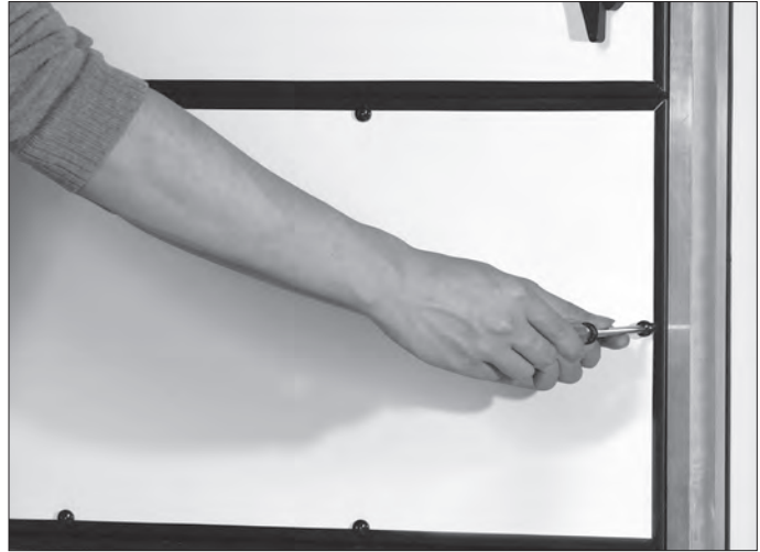
Step 1: Remove screws holding the fan access panel in place.
