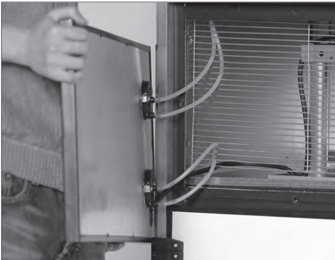
Step 3: Mark the tubes that are connected to the pressure gauges to ensure that they are returned to the correct locations later, and disconnect the tubes from the gauges.
