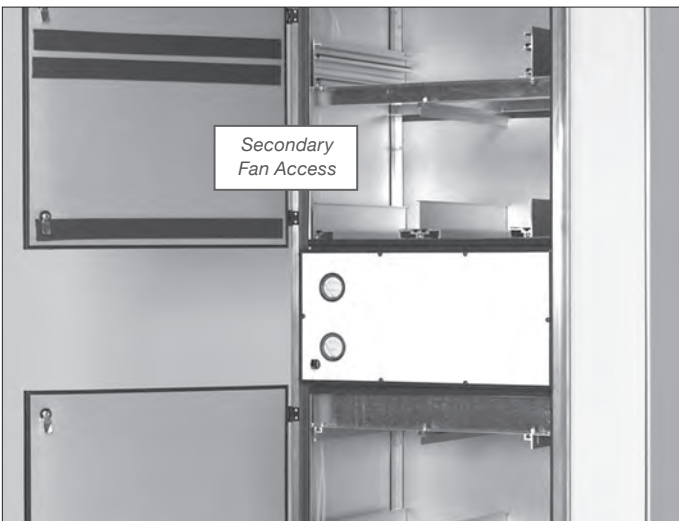
Fast but limited access to the fan can be obtained from above the fan, as shown, with the filters removed.
