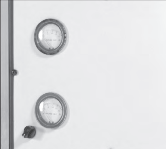
Recirculation Unit (RU) with wall mounted gauges
