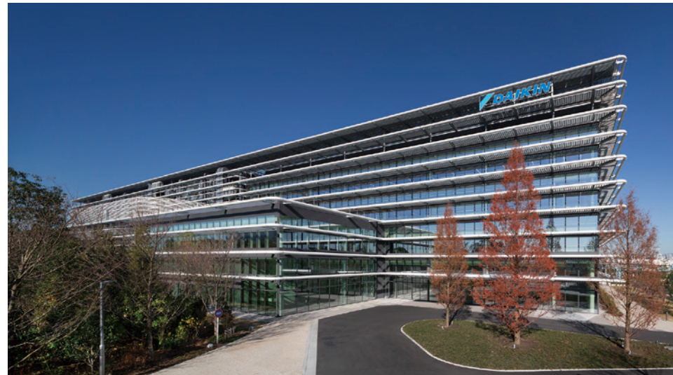
Daikin Technology and Innovation Center (TIC)
