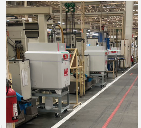
Oil Hunter™ at Customer's Plant
