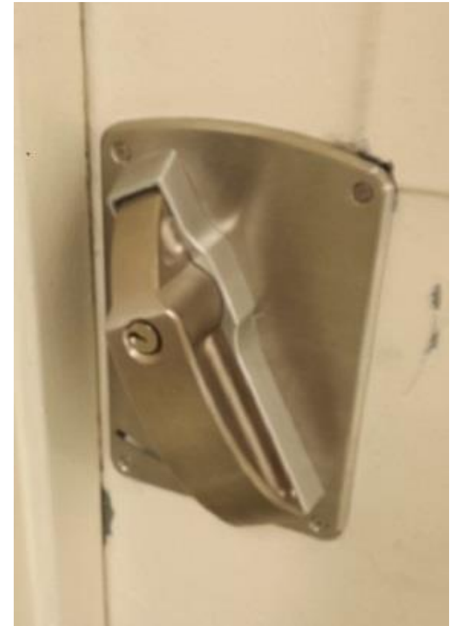
New ligature-resistant cylindrical lock
