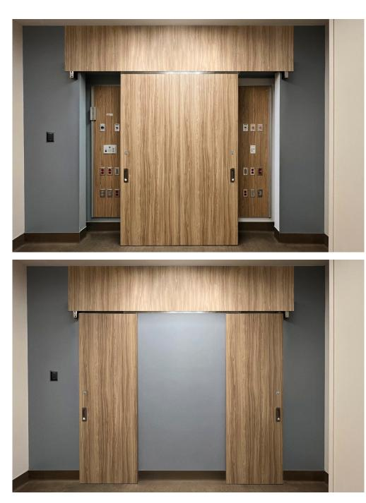
This seamless installation combines the secure cabinet design with electrified latch retraction to provide a sleek and safe solution to conceal the medical gas wall. Nursing staff presents a credential for access and then can lock the sliding door system in the open or closed position depending on the needs of the patient. All electrified components are concealed safely within the frame.
