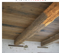
Poncer surfaces planes Sanding flat surfaces
