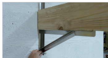
Vissage de tire-fond Screwing the lag screw
