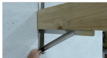
Vissage de tire-fond Screwing the lag screw
