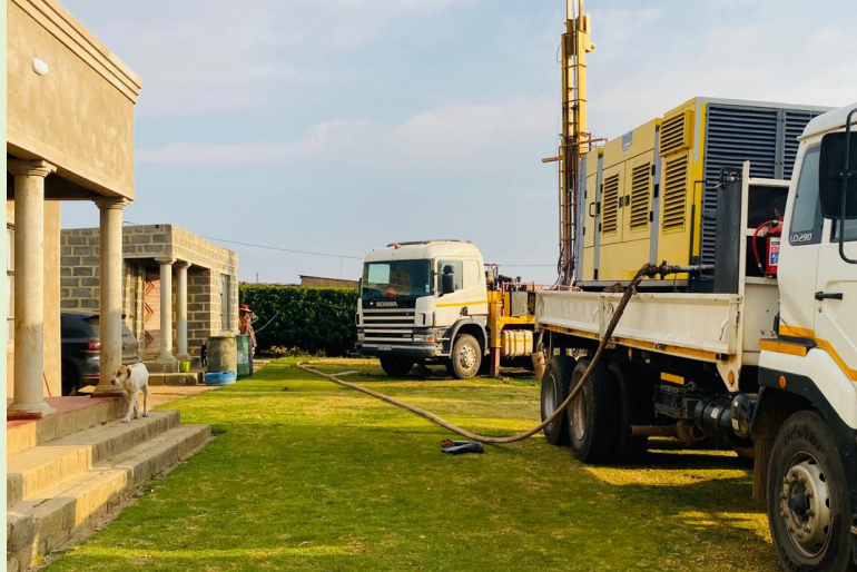
Trucks and workers on site during the borehole installation.
