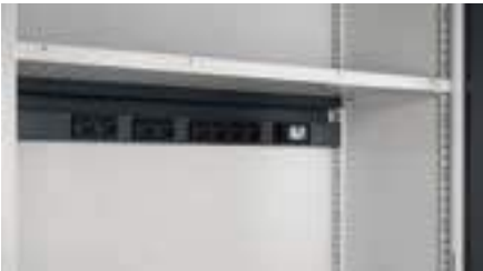
Raceway applied on the bottom part of the perforated shelf-panel
