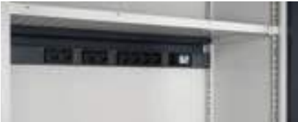
Raceway applied on the bottom part of the perforated shelf-panel
