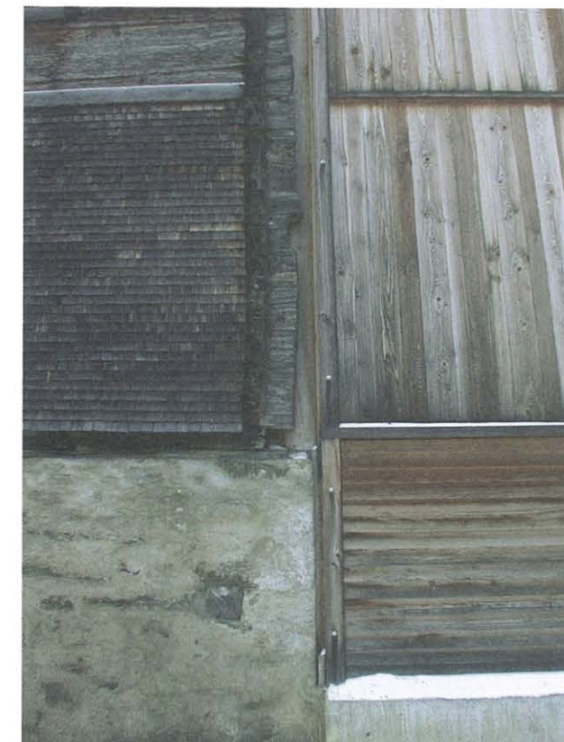
Parish hall, Vrin, original building and Caminada extension
