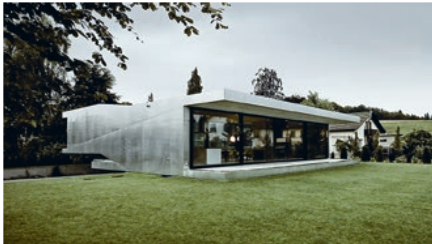
PROJECT: HOUSE FOR ONE FAMILY (2) ARCHITECT: JAN KINSBERGEN LOCATION & YEAR: LANGENTHAL (BE), 2008–2009 IMAGE: DOMINIQUE MARC WEHRLI
