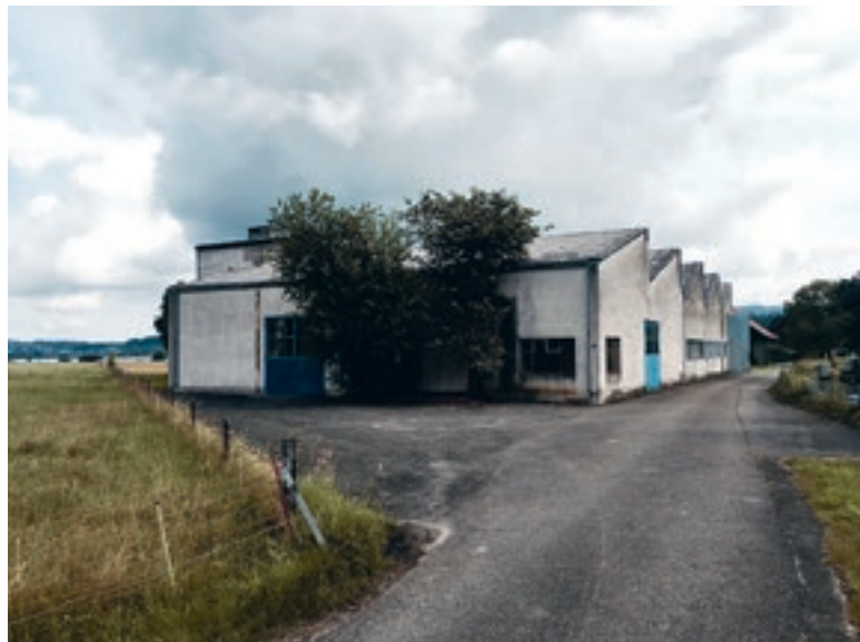
PROJECT: FACTORY BUILDING (3) LOCATION: NUOLEN (SZ) IMAGE: ALEX HURST
