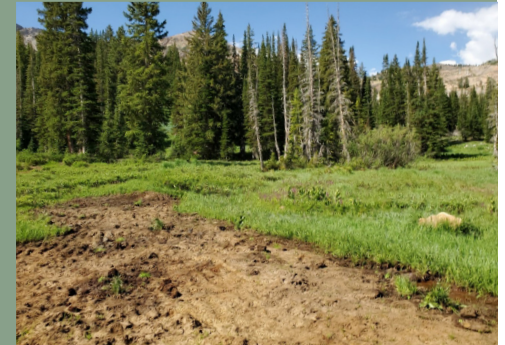
Berm removed, excavated materials used in other wetland sites July 2022
