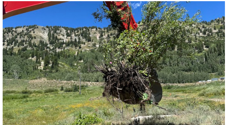
Willow relocation by root extraction with excavator
