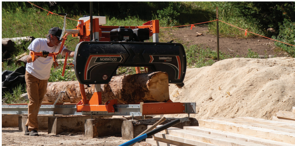
Sawmill in action—turning cut trees into reusable timber
