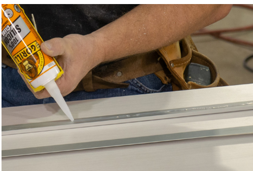
Use 100% clear silicone to adhere trim
