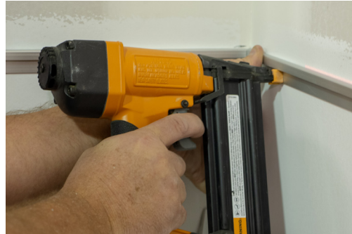
16-18 gauge 1" nails used to hold trim
