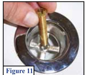
**Step 10:** Rotate the faceplate **CLOCKWISE** to the fully-closed position. Install the core guide (*Item 22*) into the strainer body using a screwdriver or 7/16" socket (Figure 11). (See core guide instruction card included with kit.) The core guide should be screwed in until it is snug against the bottom of the drain elbow. Insert the stopper (*Item 24*) into the core guide (*Item 22*) (Figure 12).
