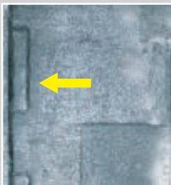
Wall reinforcement for easy installation of shower doors
