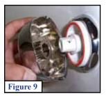
Secure the faceplate (*Item 2*) to the faceplate adapter (Figure 9) using <u>either</u> the faceplate screw (*Item 1*) (Figure 10). (Leave the plastic sleeve on threads to help align the screw.)
