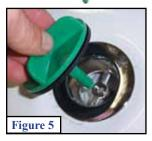
**Step 8:** After the pressure testing is complete, remove the test plug (Item 26). Cut away and discard the orange test membrane from the overflow elbow (Figure 6). Use caution not to damage internal parts on the inside of the overflow elbow.
