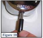
Tighten the faceplate screw until it is flush with the faceplate and snug (or if using the handle, until it is snug). DO NOT OVERTIGHTEN.
