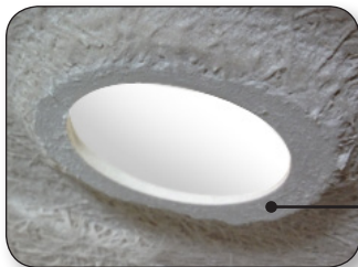
Underneath Drain View
