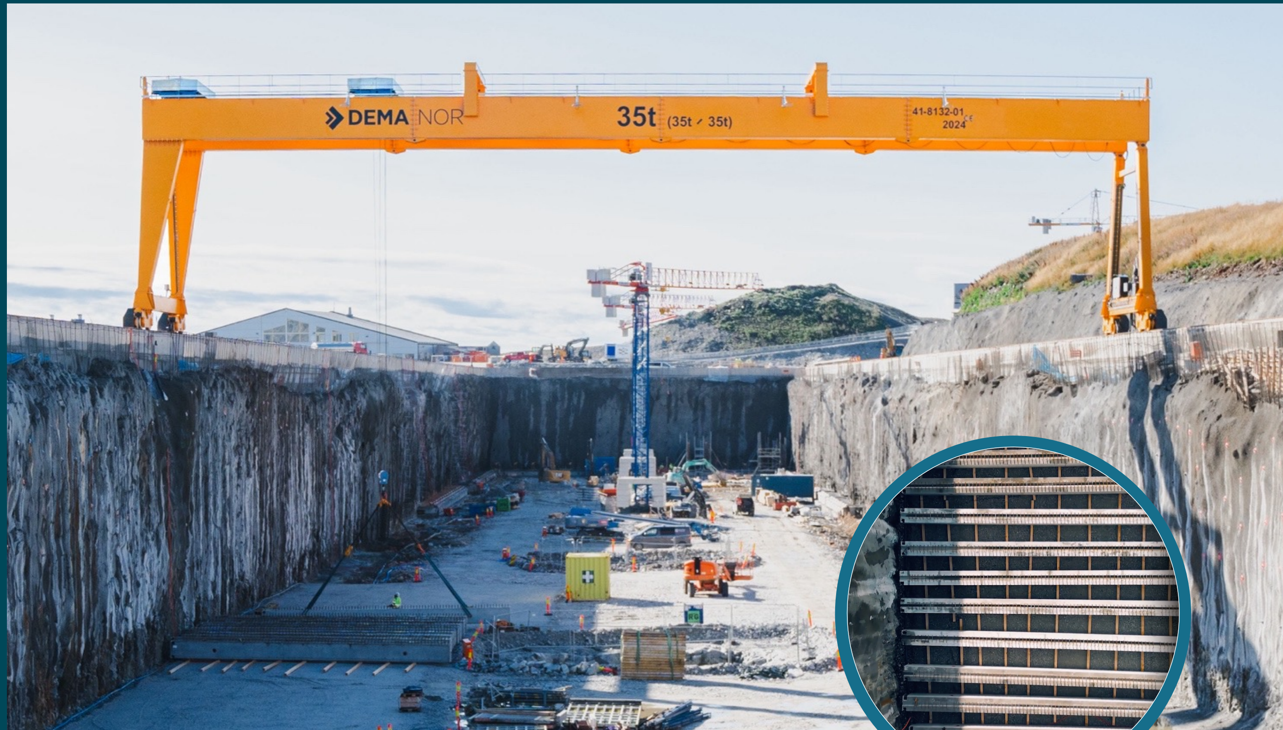
Foundation of pool floors. An on-site crane is placing concrete elements into the pool pits.
