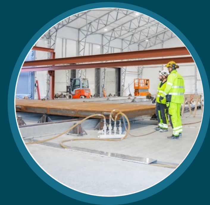
...turned into concrete elements
