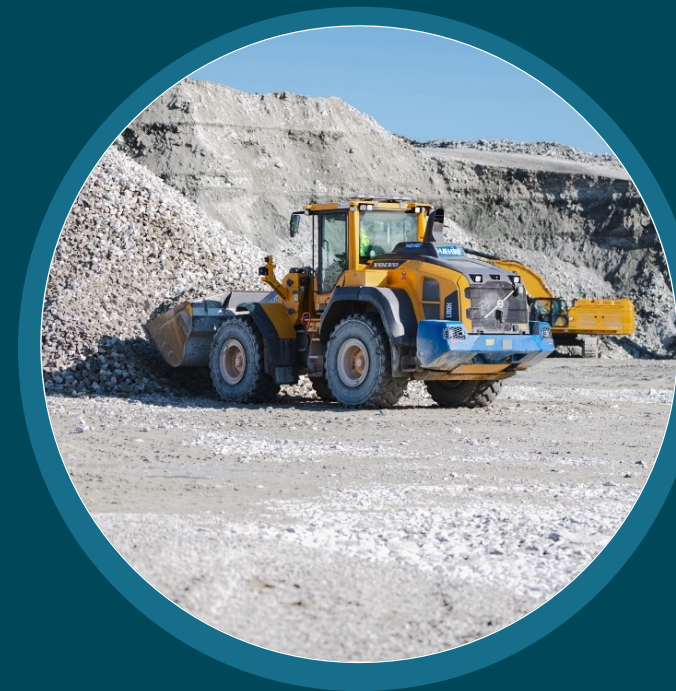
Excavated masses from pool pits...
