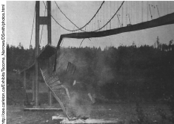
Screw-up #6: A few minutes after the first piece of concrete fell, this 600 foot section broke out of the suspension span, turning upside down as it crashed in Puget Sound. Note how the floor assembly and the solid girders have been twisted and warped. The square object in mid air (near the centre of the photograph) is a 25 foot (7.6m) section of concrete pavement. Notice the car in the top right corner.
