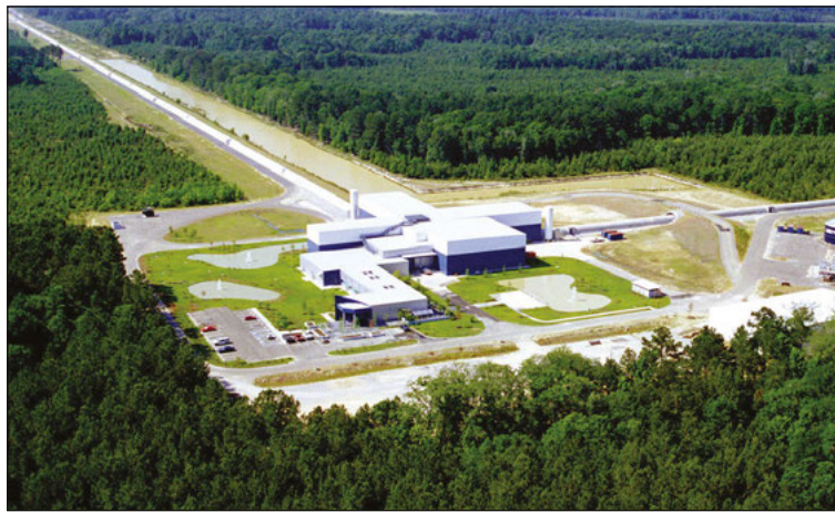
The LIGO Laboratory operates two detector sites, one near Hanford, WA, and another near Livingston, LA. This photo shows the Livingston detector site. The detector arm stretching off in the distance is 4 km long.
