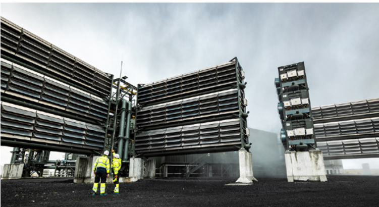
Climeworks' Mammoth plant in Iceland, which began operations in May 2024. The plant removes carbon dioxide with direct air capture — one of the methods examined in APS' latest report. Credit: Climeworks
