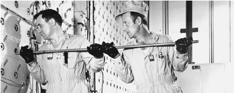
Workers used a long rod to push uranium slugs into the concrete loading face of the graphite reactor at Oak Ridge National Laboratory in the 1950s. Credit: ORNL
