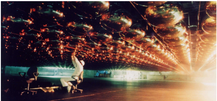
A researcher works on the Super-Kamiokande detector during construction in July 1995. Credit: Kamioka Observatory, ICRR (Institute for Cosmic Ray Research), The University of Tokyo
