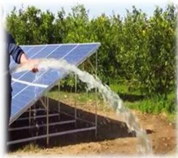
Figure 1: A photograph presenting water pumping using a photovoltaic system. (Photo Credit: The Author)
