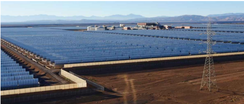
Figure 1: The Noor Ouarzazate complex, spread over 3,000 ha, comprises four solar power plants using different technologies (CSP with parabolic cylindrical mirrors/CSP with tower/Photovoltaic). The installed capacity of the complex is 580 MW. (Photo Credit: Ref. [2])
