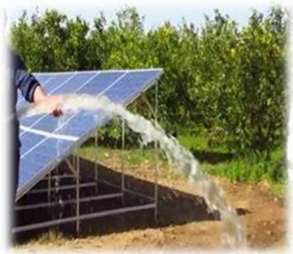
Figure 1: A photograph presenting water pumping using a photovoltaic system. (Photo Credit: The Author)
