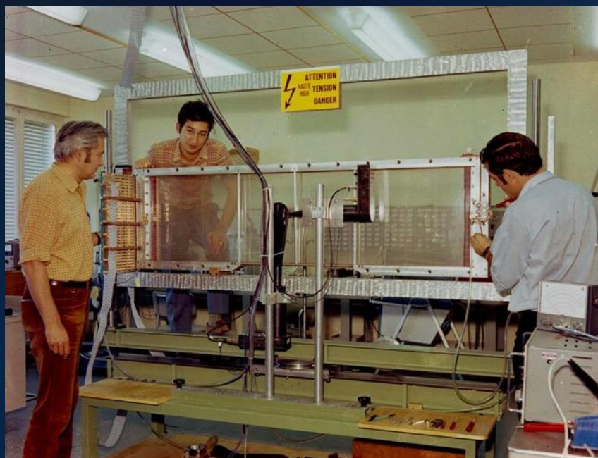
1971-1972 – Large-size Multiwire Proportional Chamber
