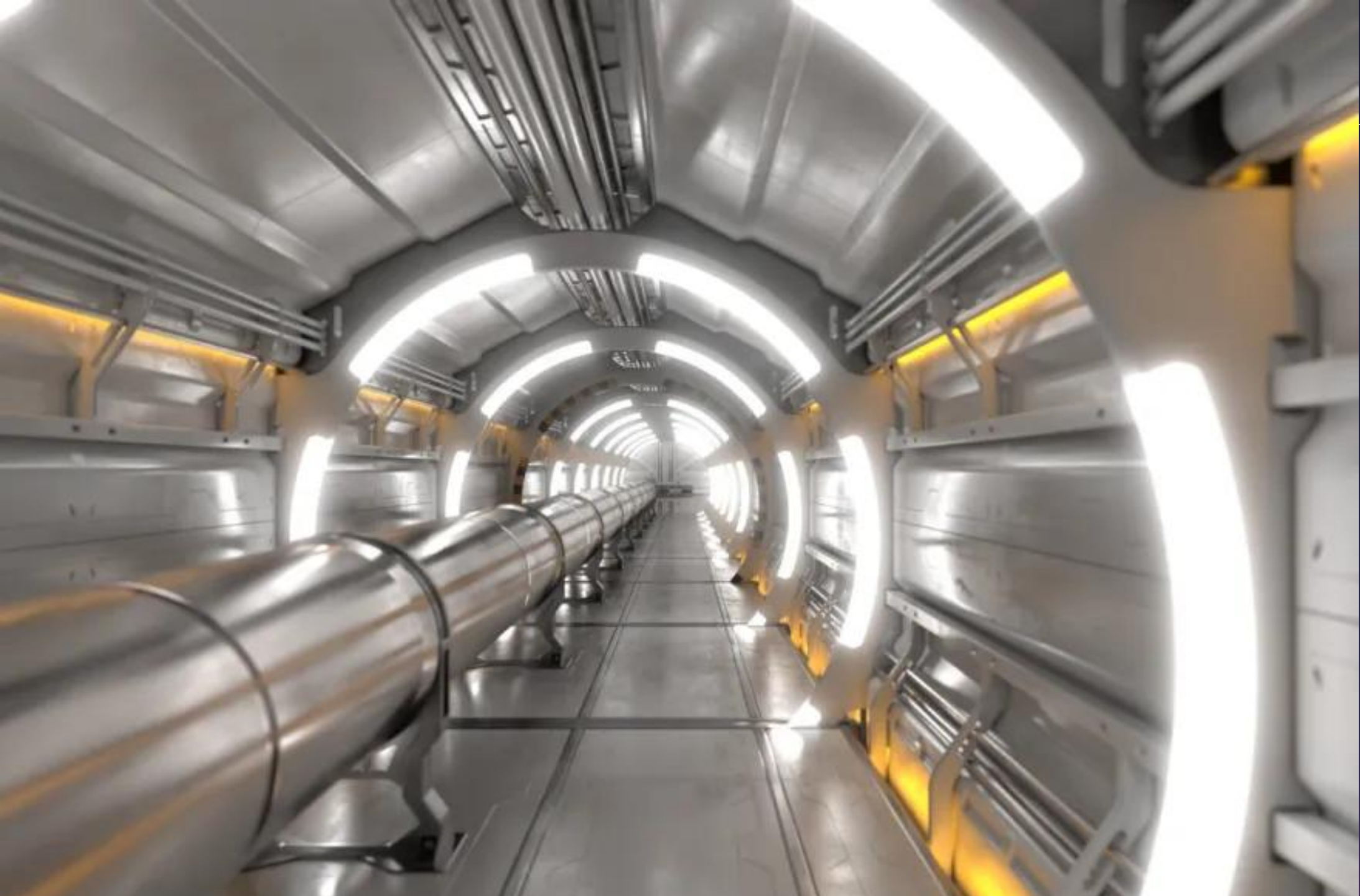
Future Circular Collider tunnel (image: CERN)
