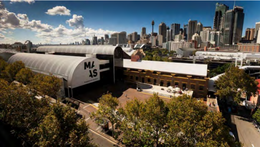
Powerhouse Ultimo, located next to Sydney CBD
