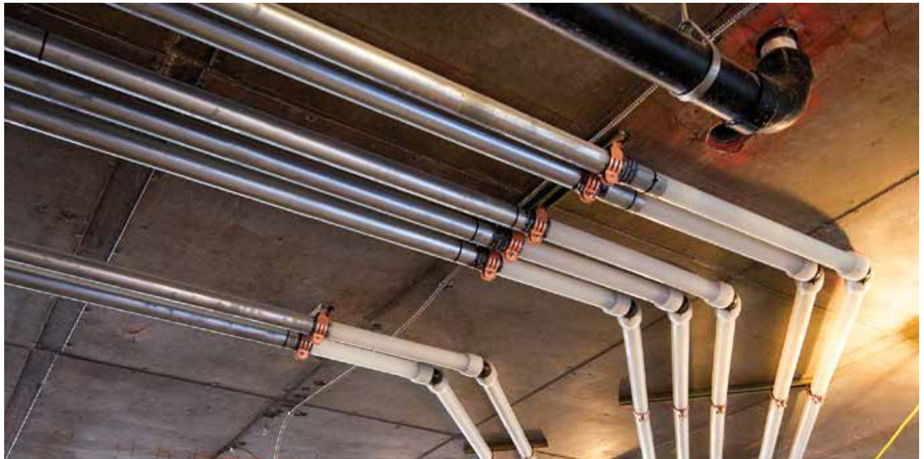
Uponor PEX-a Pipe Support installation
