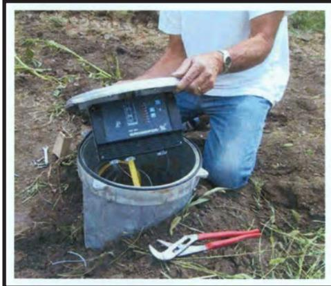
Controls mounted on plate attached to lid
