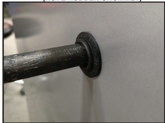
FIGURE 28 - FURNACE GAS PIPE CONNECTIONS (NOTE RUBBER GROMMET)
