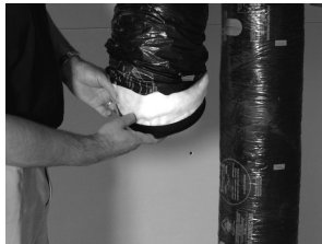
Insert insulation inside the double collar.
