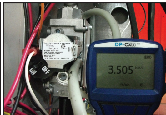
FIG. 30. - MANOMETER MEASURING GAS MANIFOLD PRESSURE
