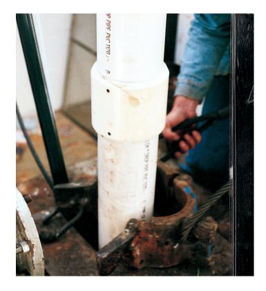
Note: As Westlake Pipe & Fittings cannot predict the degree of pump motion that may be experienced in a particular application due to factors such as mechanical unbalance, a centralizer or torque arrestor located directly above the pump should be considered, especially on deeper wells, to prevent the Certa-Lok Drop Pipe from whipping and vibrating. Use and spacing of additional centralizers above the pump should be determined based on the particular installation conditions.
