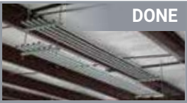
Level, tighten lock nut
