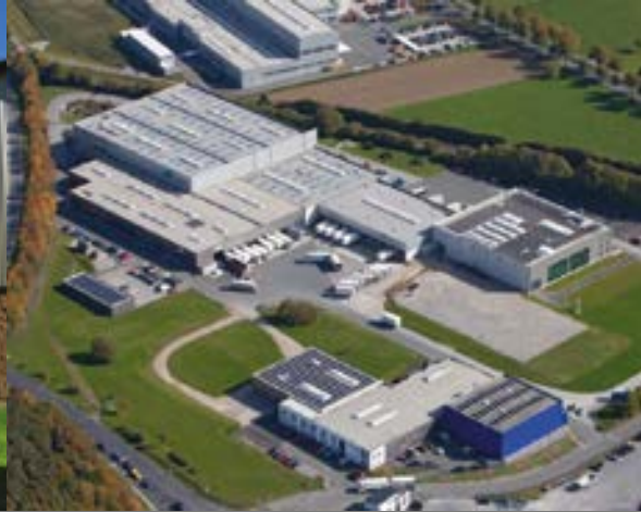
Centrotherm Systemtechnik GmbH Brilon, Germany
