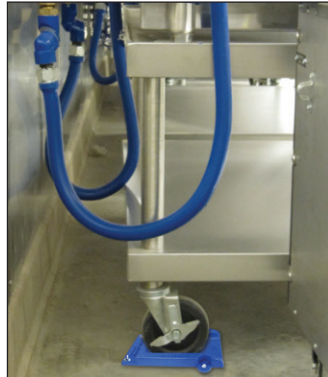
Safety-Set ensures that the appliance is situated beneath the fire suppression or ventilation systems.
