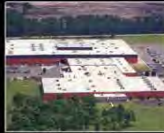
CONWAY, SC Steel Foundry and Manufacturing Plant
