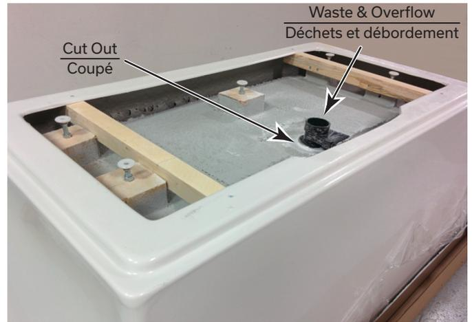
7. Lift the tub back into the correct position, levelling the tub if necessary (tub levelled at factory). Level by loosening the hex nut and threading the rod into or out of the block. Tighten the hex nut against the wood block once the foot is level. Connect the plumbing once the tub is level.
