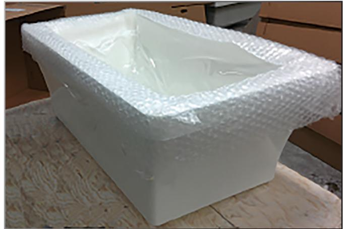
2. Position the tub in the area where it will be installed. Unscrew the drain pop-up and mark drain location.
