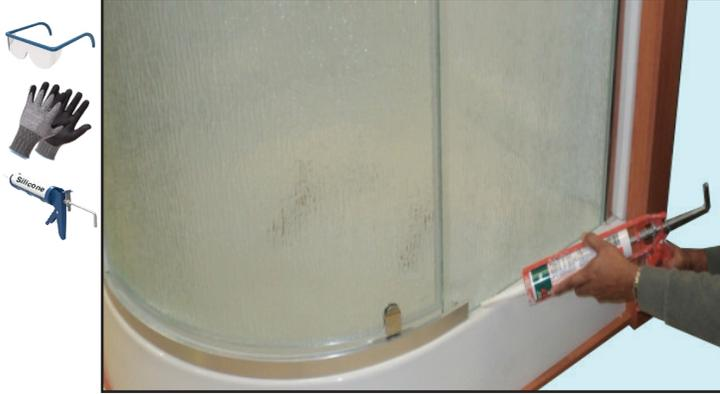
35. Finished Door Installation. If the door leaks make sure that it was sealed with clear mildew resistant silicone as specified in the installation manual.
