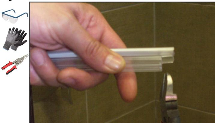
30. The Magnet Strip (10) should line up as shown. Close the door and check the magnet alignment.
