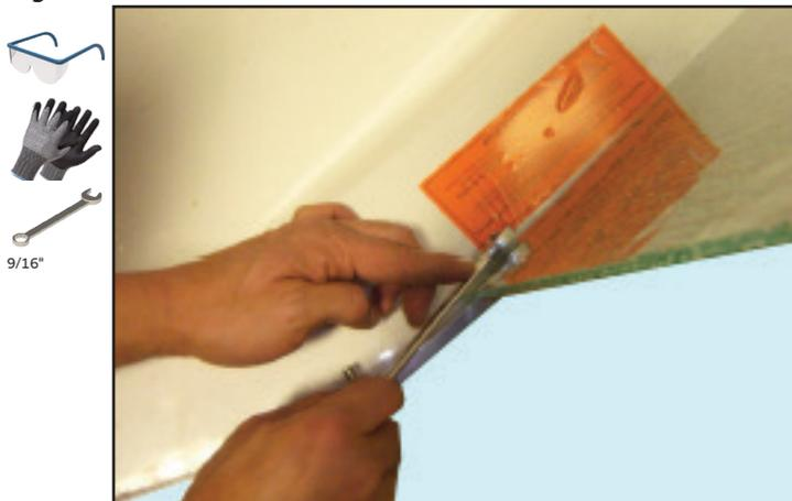
14. Repeat steps 11 and 12 for the Header (3) installation. Tighten Top Header Steel Nut (14D) snug. Reference Detail View 1 - Bolt / Nut assembly (14) on page 5 and 6 of Exploded View.
