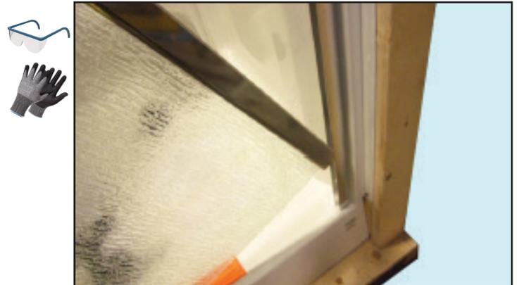
**NOTICE** Step 11 and Step 12 determine the door swing. The two door hinge studs on the sill determine the hinge side and swing of the door, Left or Right.
