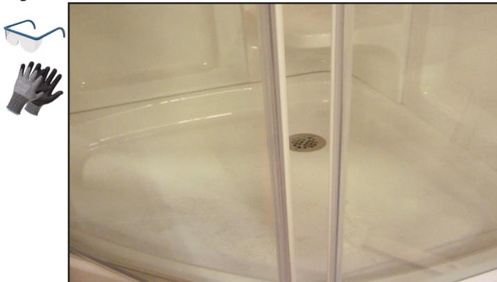
29. Notch the rigid section of the Magnet Strip (10) to match with the Bottom Gasket Seal (16) properly.
