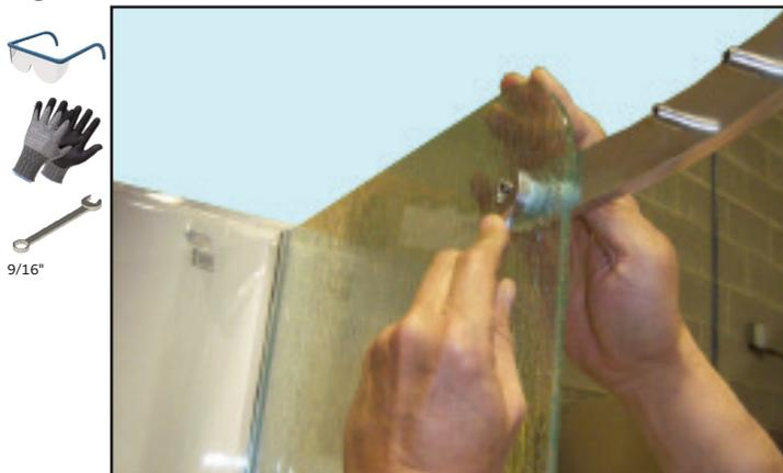
15. Place a level on the top of Header (3) to ensure that the Header (3) is level, then tighten nuts.
