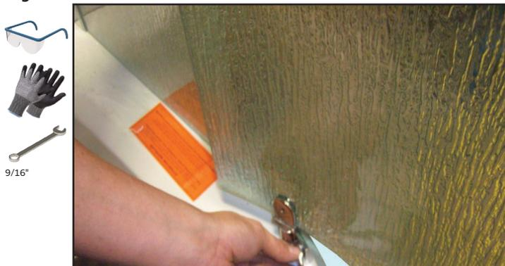
32. If the Magnet Strip (10) is not closing tight: Use a piece of wood, tap the wood block with a mallet to adjust and align the magnet seals in the areas required.
