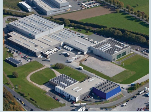
Centrotherm Systemtechnik GmbH Brilon, Germany
