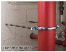
Integrated second set of bolt holes allow the assembly to easily adapt from a riser clamp into a stand-off support
