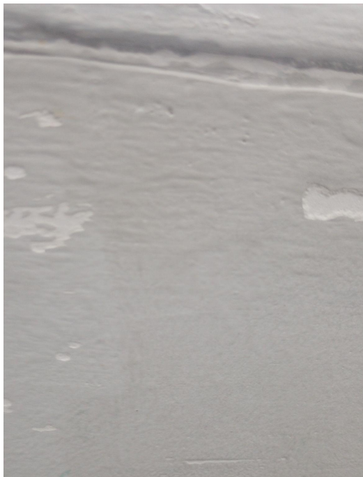
Chipped paint on various areas on the living room walls in the apartment home
