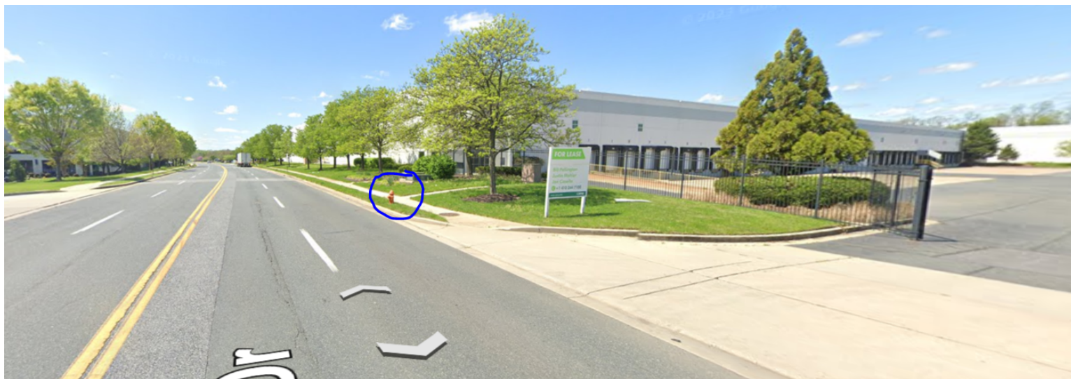
8416 Kelso Drive - gushing fire hydrant 8/8/25
