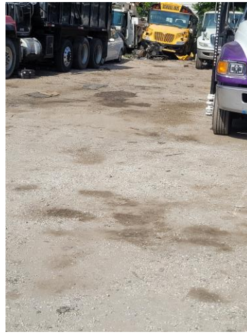
Apparent oil stains on ground
